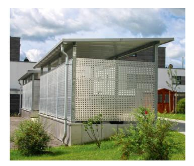
The trapezoidal sheet is used for the economical design of roofs. The galvanised rolled section, made from steel, is coated with protective lacquer on one side, while the other side gets a powder coating which is available in a variety of RAL colours.
